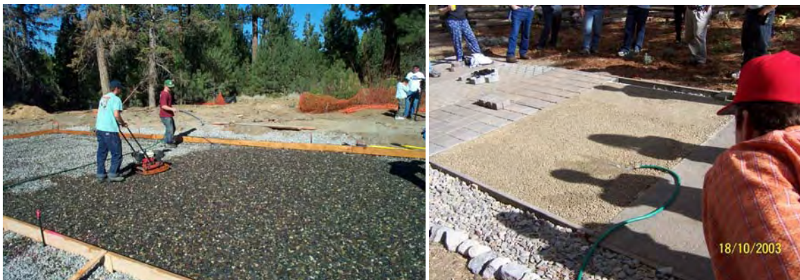
Figure 3-23. Demonstration project at Lake Tahoe. Underlying clean gravels being installed (left) and water rapidly infiltrating into porous concrete (right).
