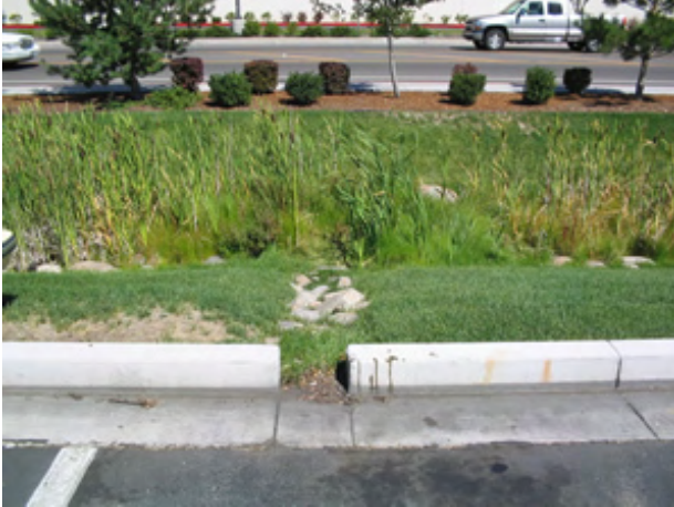
Figure 3-43. Curb cuts direct water into this parking lot bioretention system.
