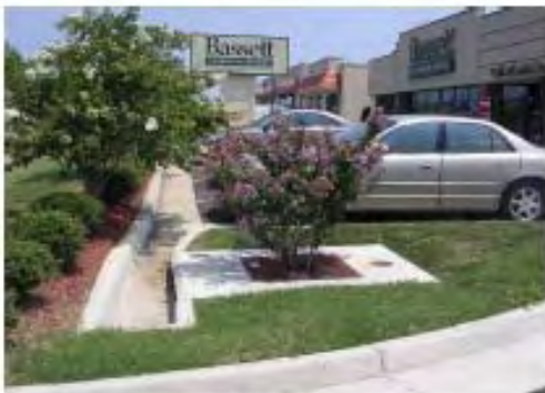
Filterra used with a flumed bypass in a commercial parking lot.
