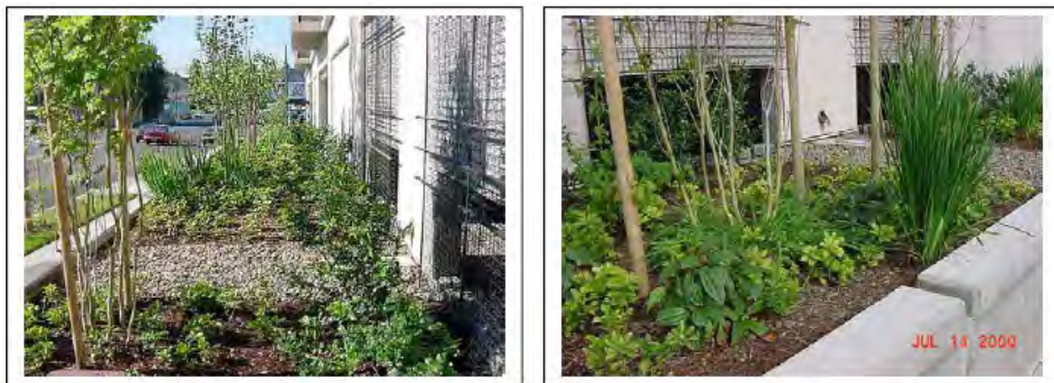
Figure 3-18: Storm water planters installed next to office buildings. (Source: Portland BES)
