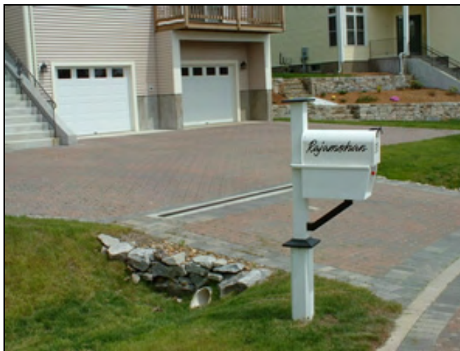
Figure 3-47. This driveway is designed with multiple LID strategies including permeable pavers and a slotted drain built in to catch sediment and runoff, which is funneled into a landscaped area. (Photo courtesy of NEMO Nevada )
