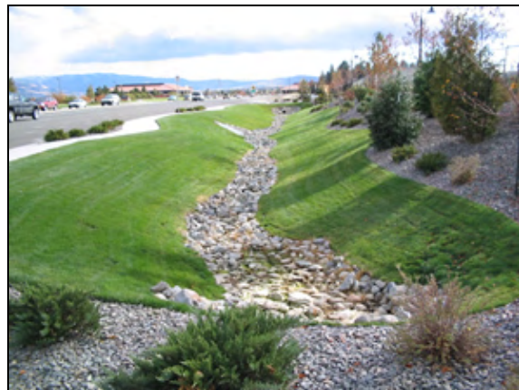
Figure 3-20. Swale with rock lined low flow channel
