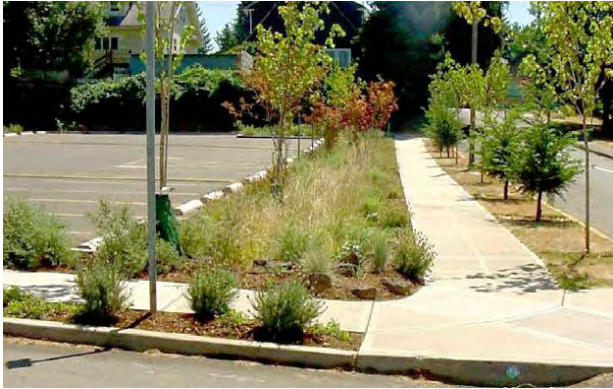
Figure 3-7: Landscape detention basins located at the edge of a parking lot (left photo) and in a parking lot island with turf and shrubs and trees (right photo).
