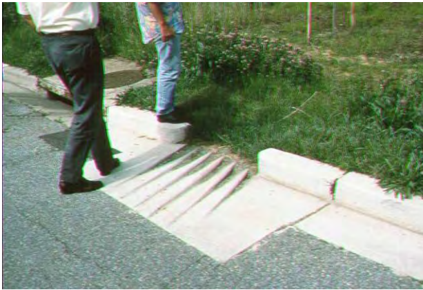
Figure 3-8: Curb opening design for a landscape detention system located upstream of a conventional storm drain inlet (left photo). A bioretention system retrofit into an existing parking lot island (right photo).
