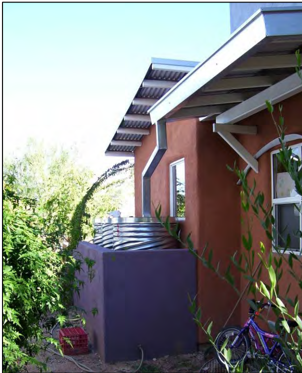
Figure 3-28: A rainwater catchment system on a residential home. (Photo: Kennedy/Jenks Consultants)
