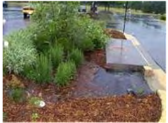
Figure 3-8: Curb opening design for a landscape detention system located upstream of a conventional storm drain inlet (left photo). A bioretention system retrofit into an existing parking lot island (right photo).
