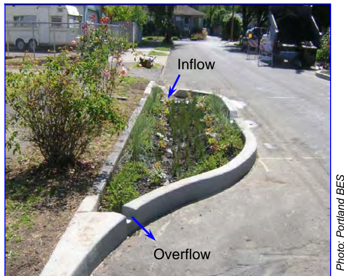
Figure 3-6: Bioretention system incorporated into a traffic calming feature with inflow and overflow through curb openings.
