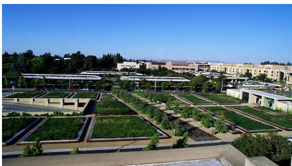
Figure 3-35: Intensive Green Roof on a parking structure at Stanford University, Palo Alto, California.
